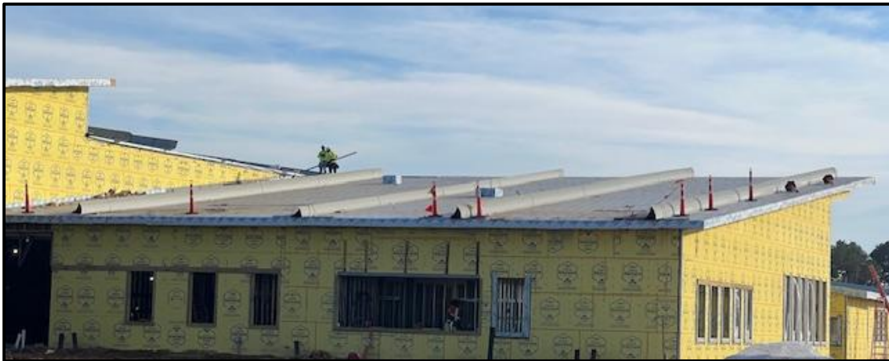
Metal Panels at Roof
